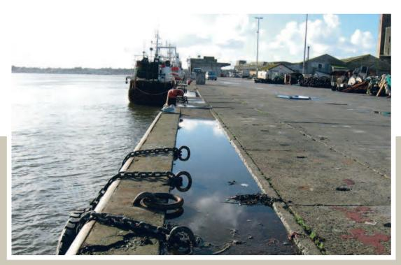
Natural cement allows the rapid return to use in the short term, even in cold weather.
