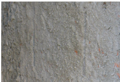
Preping the substrate with rough cast
